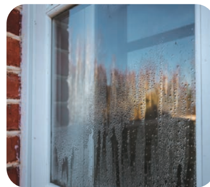
Misted Units Replaced
